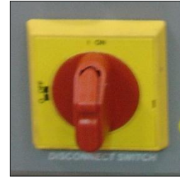
Figure 1. Disconnect Switch.
